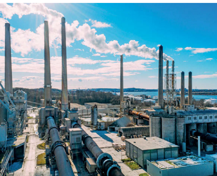
Aalborg Portland's cement kilns emit around two million tonnes of carbon dioxide per year Source: Aalborg Portland Holding
